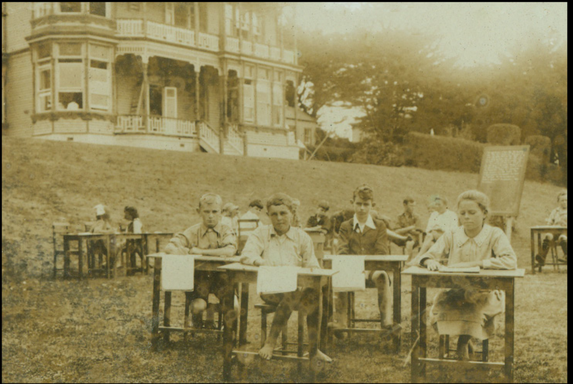
1919 Lessons outside Vasanta House
